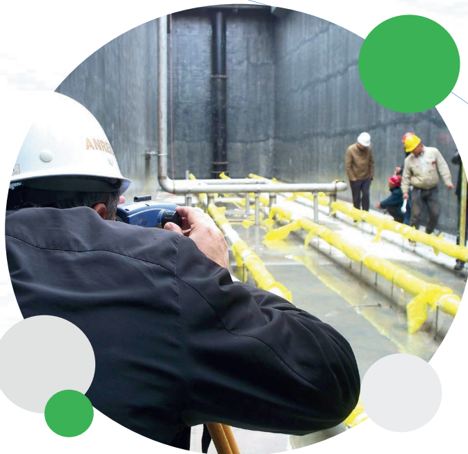
SHANYIN, CHINA (Installation of ESMIL Aeration System)
