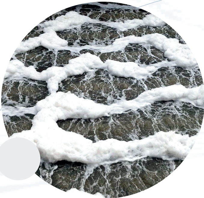
HULAN DISTRICT, HARBIN, CHINA (Installation of ESMIL Aeration System)
